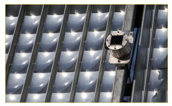
Tracking system with solar camera
